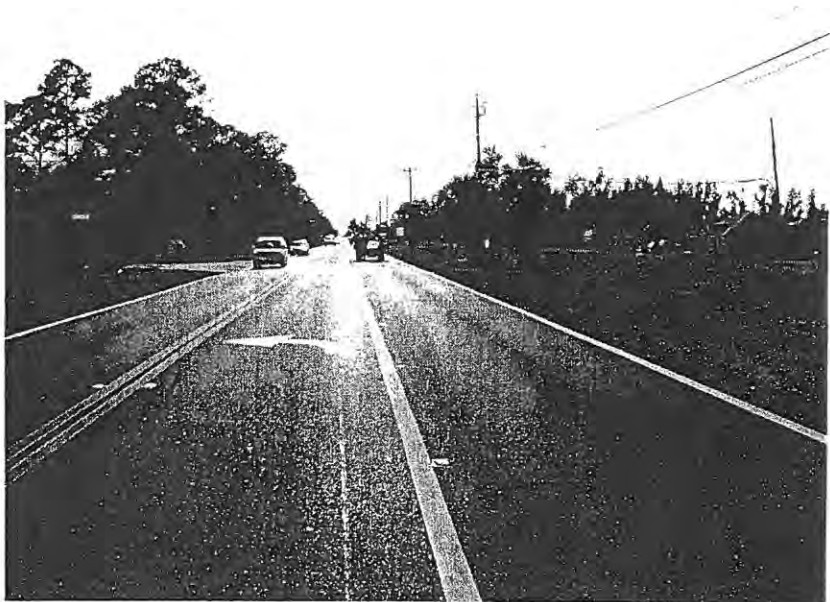
Malabar Rd WB Approach to Garvey Rd
